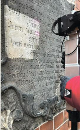
Laser cleaning is an advanced process where the precise selection of equipment and laser beam parameters plays a key role. During cleaning, ablation occurs. Appropriate wavelength and optimal process parameters enable laser radiation to be absorbed by surface contaminants. After the particles adhering to the substrate are detached, the laser radiation does not penetrate deeper into the material, enabling cleaning without significant interference or surface damage.
